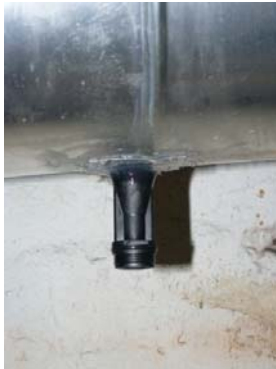
Collector Funnel secured in place using a standard silicon sealant
