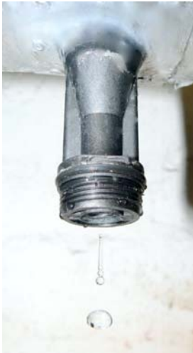
This picture clearly shows fluid exiting the collector funnel from within the insulated pipe
